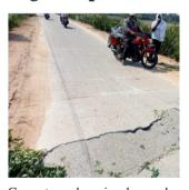
Concrete road causing damage by heavy temperature due to expansion. Now the damaged road causing problem communication. People demand a high lebel enquary by technical team. This road work completed just before one month and damaged within one month due to negligency of RD Department.
